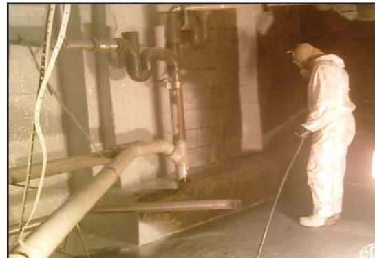
Applying ARC S1HB by heated plural component spray
