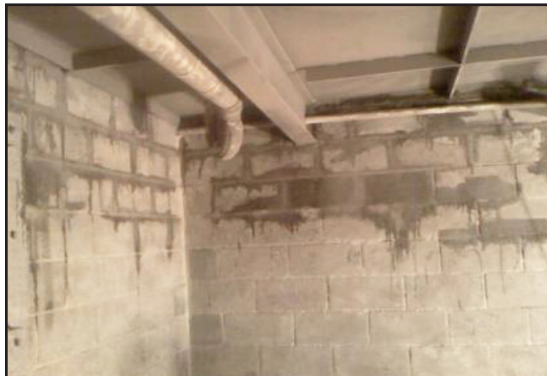
Water blasting and grout patched concrete
